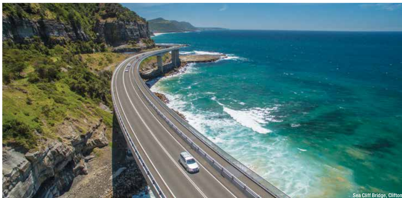
Sea Cliff Bridge, Clifton
